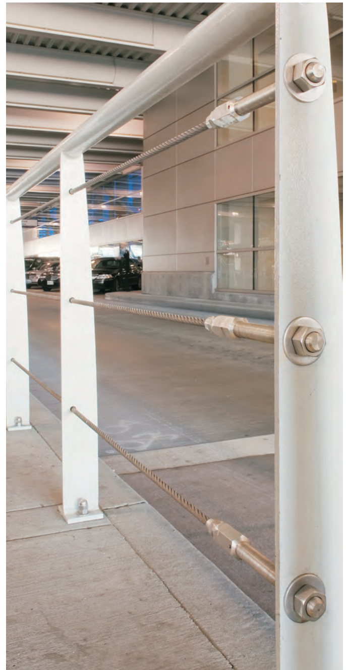
Stud Fitting - Pedestrian Walkway - Portland International Airport
